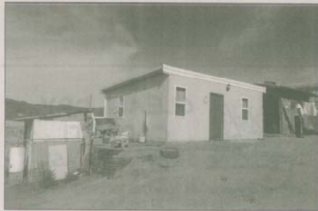
SUBMITTED PHOTO Simple, easy-to-assemble homes like this one are being manufactured for poor residents of Mexico. The homes feature materials made by Cordeck, a Kenosha company.
